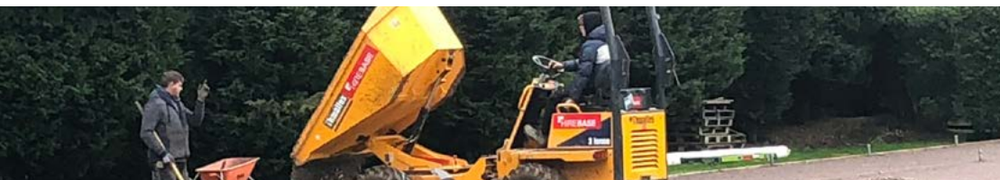
Practice Net Restoration project, West Bromwich Dartmouth Cricket Club (WBDC)
